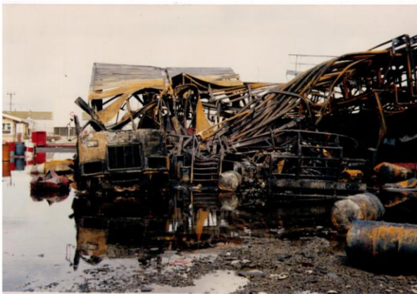
Truck loading area after the event
